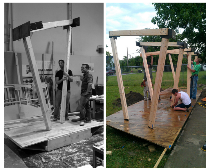
Figure 5: full-scale prototype (left), bolting the structure together on site
